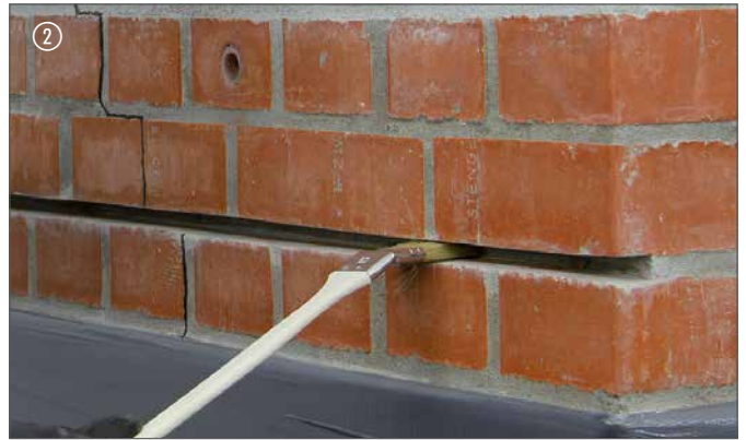
Fuge reinigen | Clean the joint / slot
