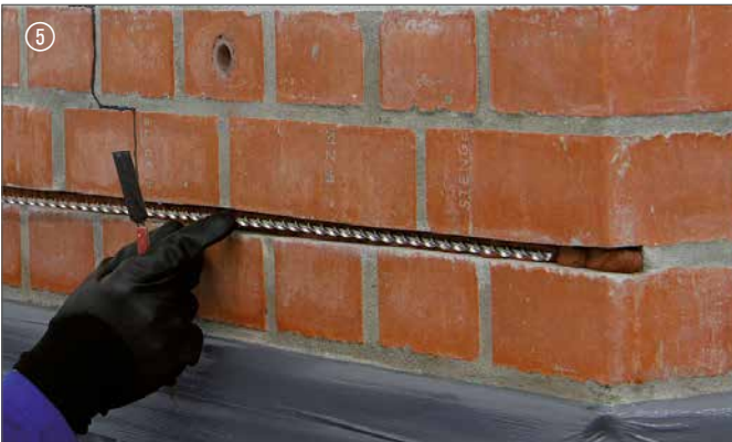
Spiralanker setzen | Place the spiral anchor
